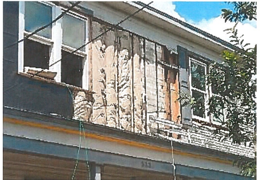
Insulation and wood windows in enclosed second floor porch.
