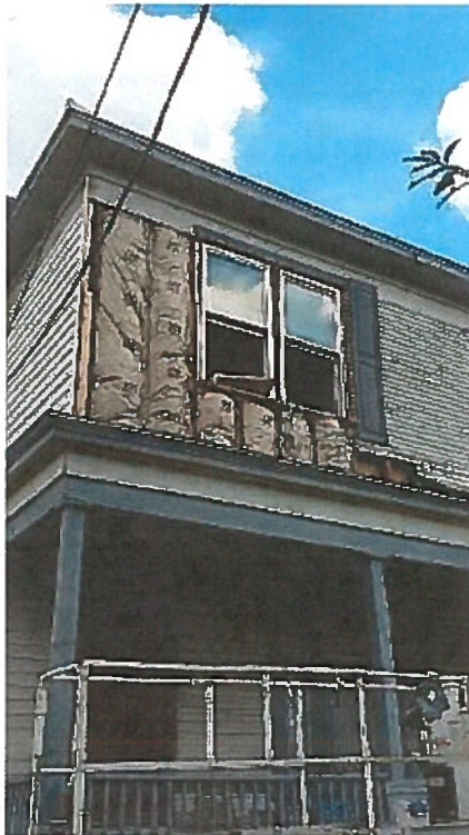
Insulation and wood windows in enclosed second floor porch.
