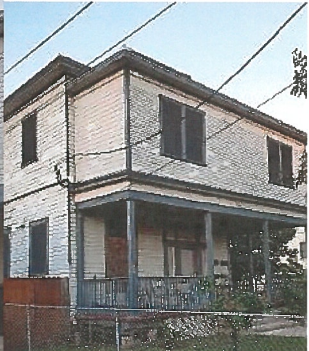
Exterior repaired with insulation, siding, windows (repaired/replaced) as approved by Historic Preservation Commission. This included removal of the east facing window in the enclosed upstairs porch near the electrical power line.
