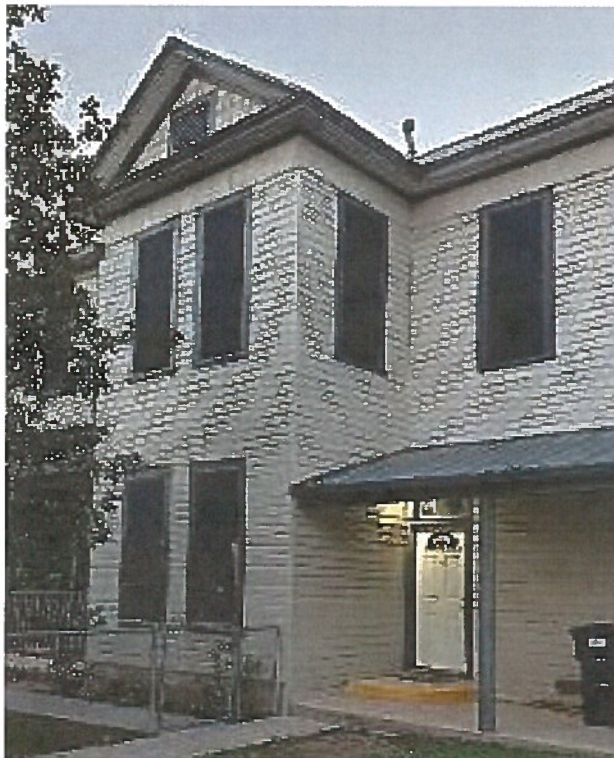
Exterior repaired with insulation, siding, windows (repaired/replaced) as approved by Historic Preservation Commission. This included removal of the east facing window in the enclosed upstairs porch near the electrical power line.
